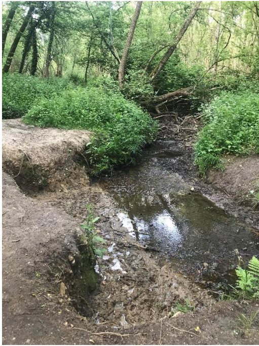
Picture 2 one of the areas of deterioration along the stretch of River bordering the green
