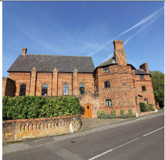
Figure 8 The Former Hautboy Inn, Ockham
